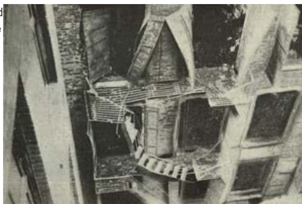
Fire escape of Asch building after the Triangle fire, New York City, 1911. Photo courtesy of the Library of Congress.
